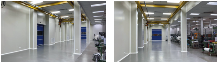
New section of cleanroom 1 after upgrade completion
